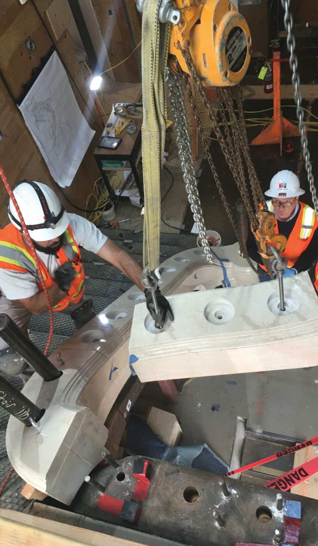
QuarryHouse built an overhead crane system and hung it from ceiling beams. Here the crew is placing one of the stair bases. Then, they’ll insert steel rods on which to place the balustrades. Photo courtesy of QuarryHouse
